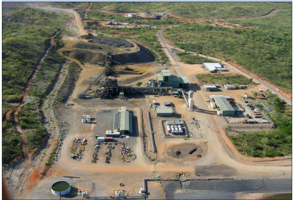
Fig. 2: Savannah Plant Infrastructure
